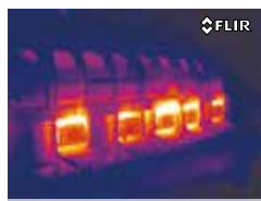
Refractory insulation defect
