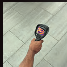
Check floorheating for leaks
